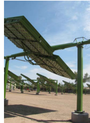
Solar at Water Treatment Facility City of Somerton
