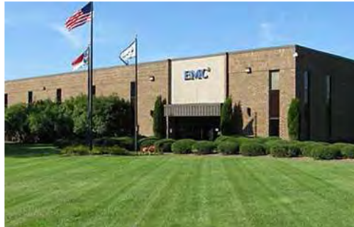
EMC's facility in Apex, N.C. photo courtesy of EMC
