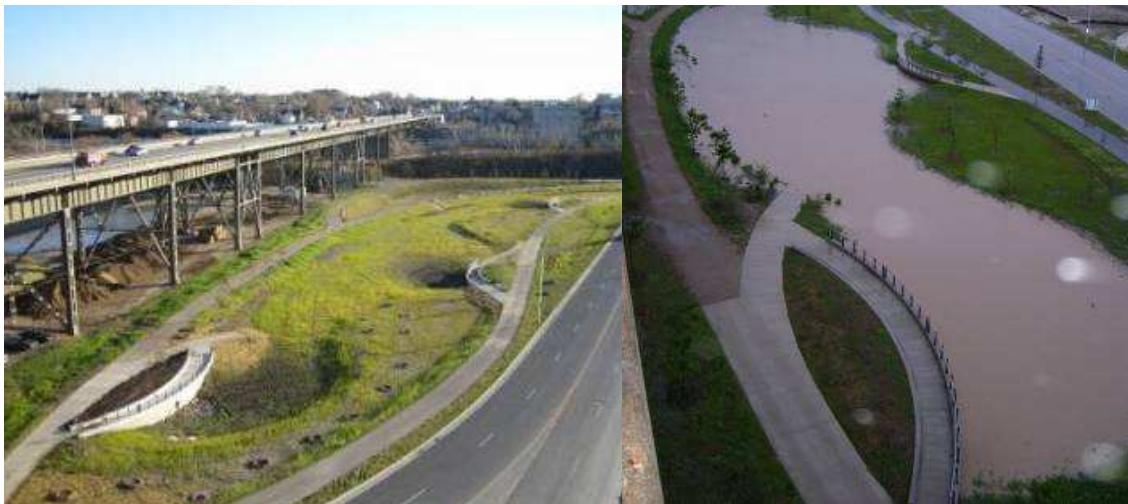
Floodable Park dry (at left) and after a 2008 100-year storm (at right). Printed with permission from MVP. Photo credit: Menomonee Valley Partners, Inc.
