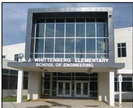
Figure 5: A.J. Whittenburg Elementary School of Engineering. [Source: http://www.greenville.ks12.sc.us/ajw/about/contact.asp ]
