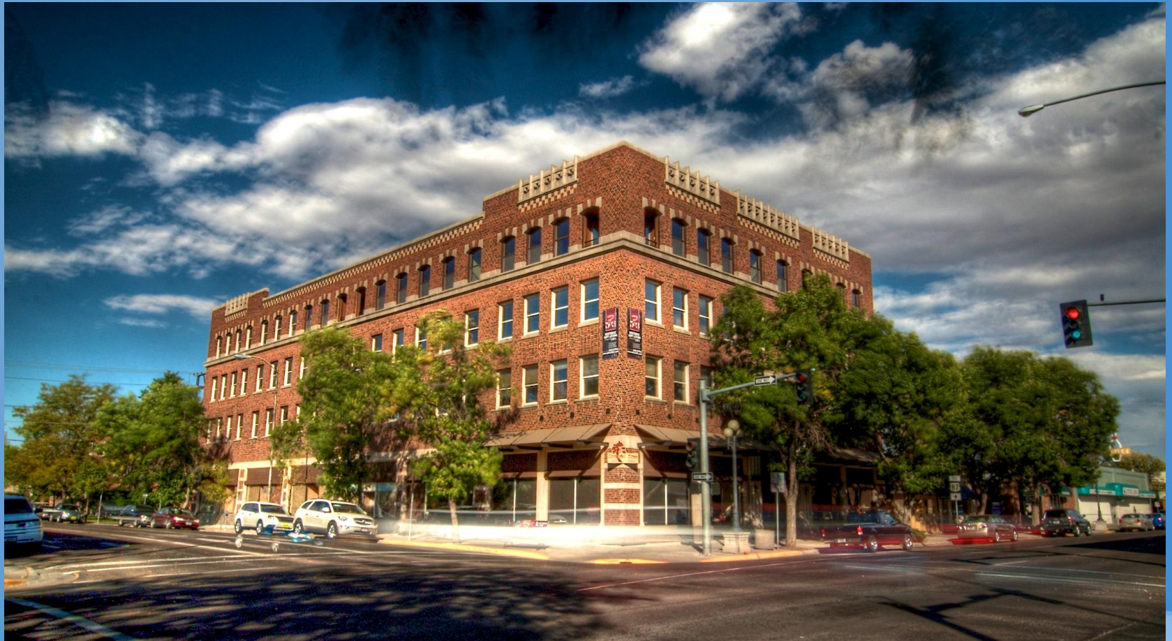
Montana Building, Downtown Great Falls
