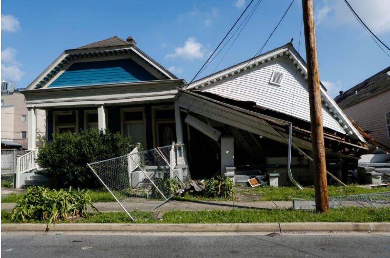
Damage from Hurricane Ida in New Orleans in September 2021. After four hurricanes in two years and 11 insurer insolvencies, the Louisiana Insurance Guaranty Association is turning to the bond market. Bloomberg News
