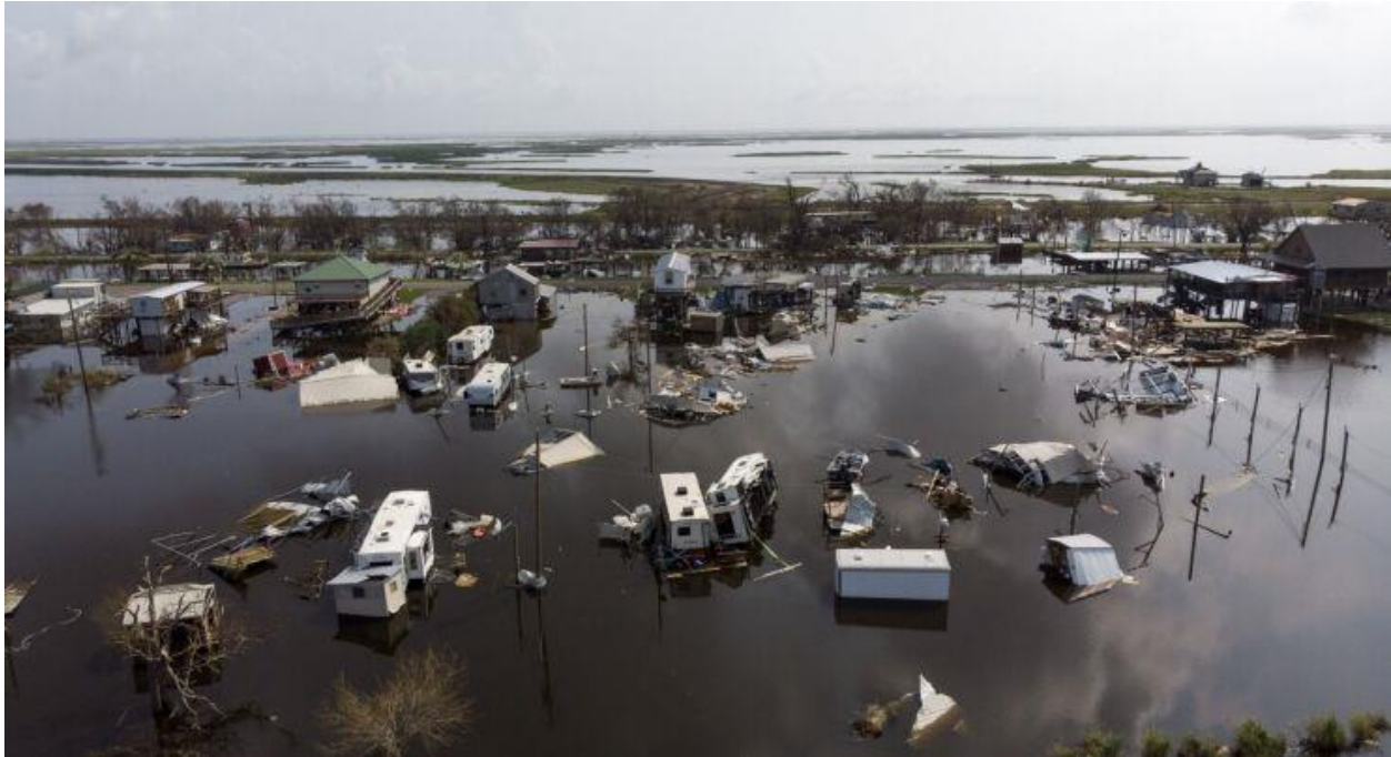
Damaged homes in Pointe-Aux-Chenes, Louisiana, sit in flood waters after Hurricane Ida hit in September 2021.
