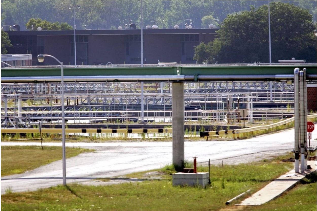
The Metropolitan Water Reclamation District of Greater Chicago's Stickney Water Reclamation Plant. Bloomberg News
