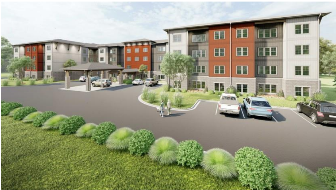
A rendering of the Flats at Mt. Zion in Clayton County, Georgia, which are being developed with the help of tax-exempt bonds. KeyBanc Capital Markets
