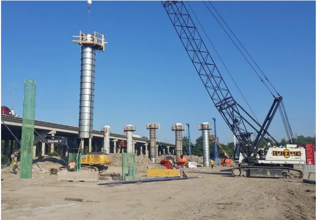
Bridge construction on Interstate 294 in August as the Illinois State Toll Highway Authority works through a $14 billion capital program. Illinois State Toll Highway Authority
