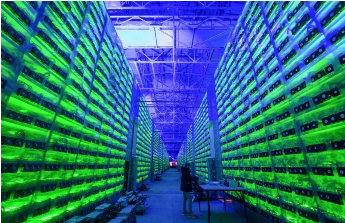
A worker inspects computer rigs in a cryptocurrency mining farm in Russia in March. Massive computing power, and associated power consumption, is required to create and maintain the blockchain ledger. Bloomberg News
