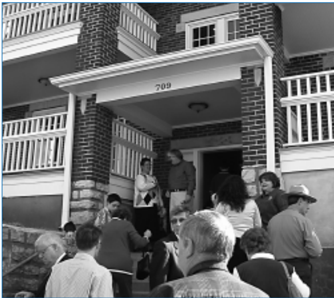
Patriot Place Apartments, LLC, used state and federal historic rehab tax credits and funding from the National Trust Loan Funds to rehabilitate a fire-ravaged apartment building in the Harry S. Truman National Historic Landmark district in Independence, Mo. The project produced 17 apartment units, including 10 reserved for low- to moderate-income renters. Photo by Lisa Weissman.
