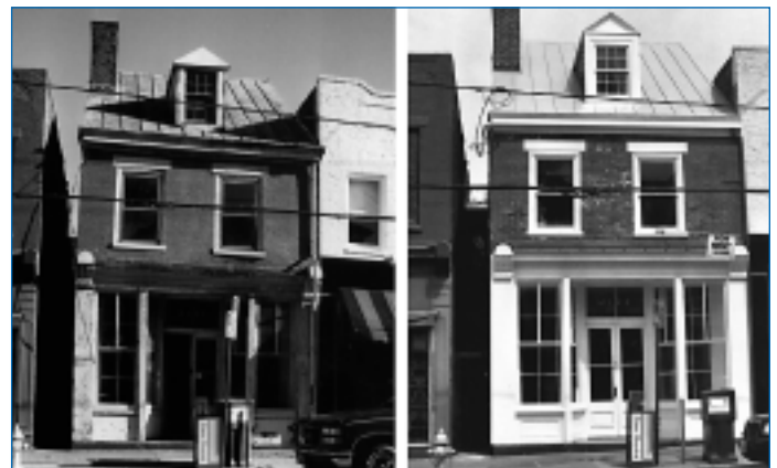
Property owners in Virginia can take advantage of a 25 percent state tax credit for rehabbing a National or state register property. Pictured above is 2114 East Main Street in the Shockoe Valley and Tobacco Row Historic District located in Richmond, Va. Photo courtesy of the Virginia Department of Historic Resources.
