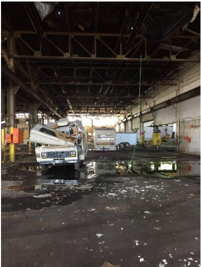
Figure 2: Interior view of main building, which is currently used for storage.
