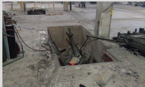
A demolition crew member works inside the escalator pit.
