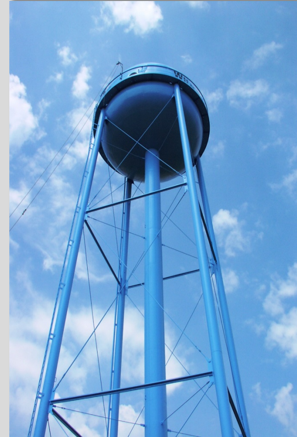
Winesburg Water Improvement Project Holmes County
