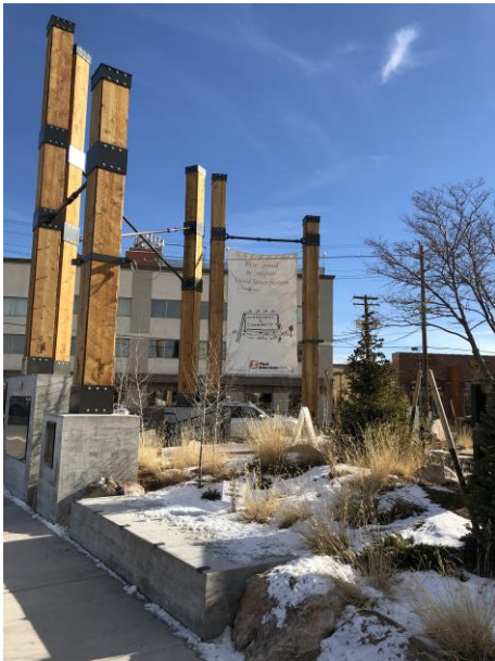
David Street Station in Downtown Casper
