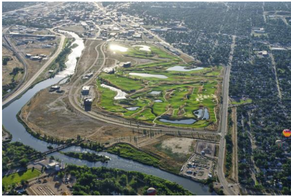
Casper Redevelopment Site
