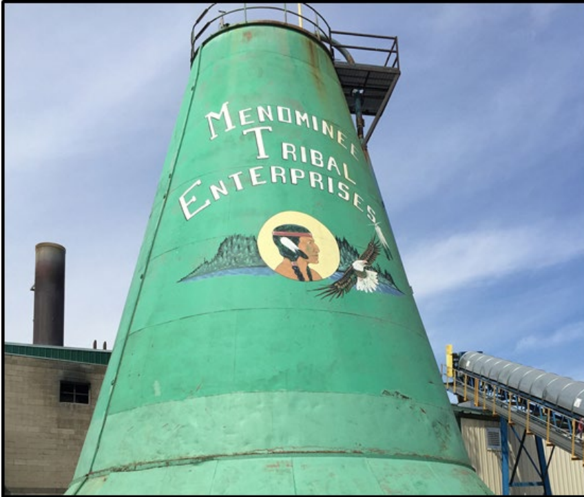
Menominee Tribal Enterprise (WI) Ribbon cutting for biomass combined heat and power system (April 2016)
