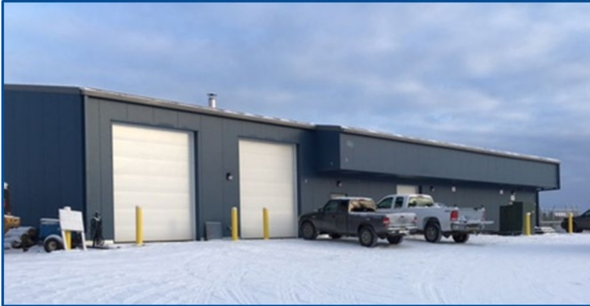
Council Of Athabascan Tribal Governments and Gwitchyaa Zhee Corporation (AK) Combined Heat and Powerhouse (below) and the Old Power Plant (top) (December 2017)
