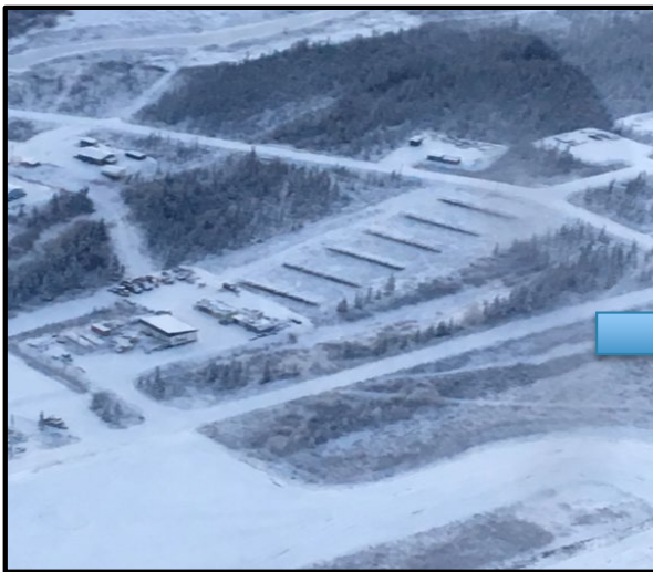
Future Site of Hughes Solar PV Array (AK)
