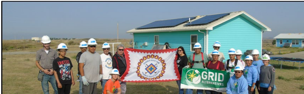
Rosebud Sioux Tribe (SD) installed a solar system on low-income home (August 2016)
