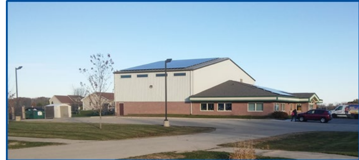
Oneida Nation (WI) installed 800 kilowatts of solar photovoltaic for 6 buildings (November 2017)
