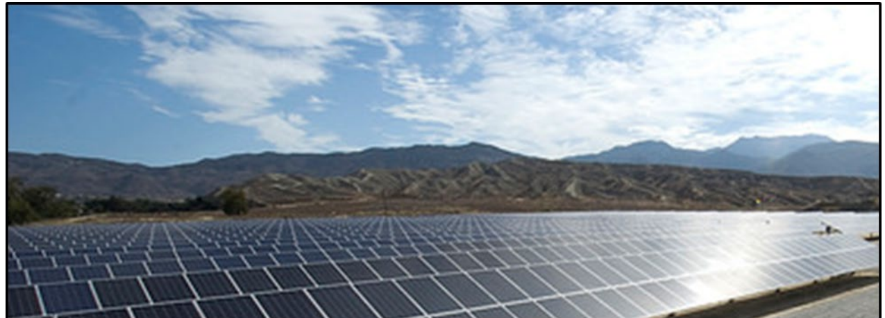
Soboba Band of Luiseño Indians (CA) 1 MW solar installation (July 2016)
