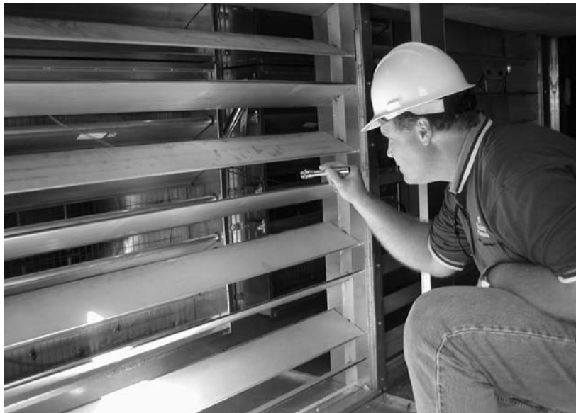
Wiley & Wilson employee inspects an air handling unit.
