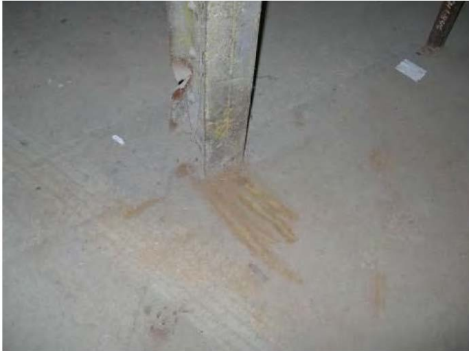
Photograph 7. Looking at one of the locations sampled for the SSD04 surface soil sample in the northern portion of the Fintube Building
