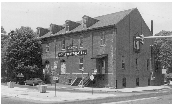
Edward McGovern Tobacco Warehouse. Lancaster, Pennsylvania (ca. 1880). Rehabilitated for commercial use. Courtesy: Michael Oehrlein. Photograph: Historic Preservation Trust of Lancaster County.
