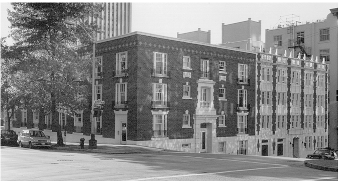
Pacific Hotel Apartments (historic name: Leamington Hotel and Apartments), Seattle, Washington (1915). Rehabilitated to provide 112 units of housing for low income and homeless people. Courtesy Stickney & Murphy. Photograph: Mike Romine.
