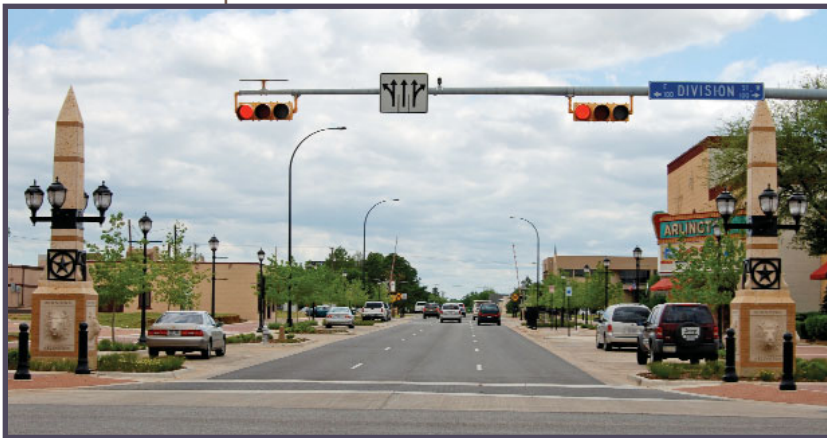
Center Street streetscape improvements
