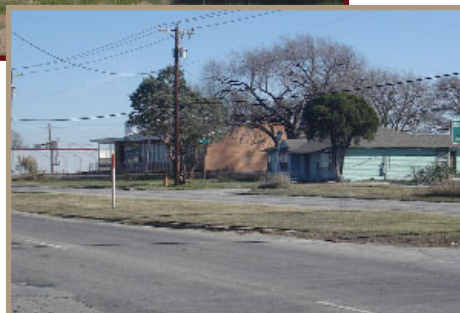
Existing structures along Abram Street
