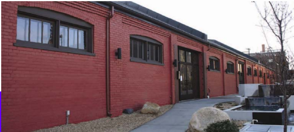
RICHMOND, VIRGINIA CRAWFORD MANUFACTURING COMPANY BUILDING
