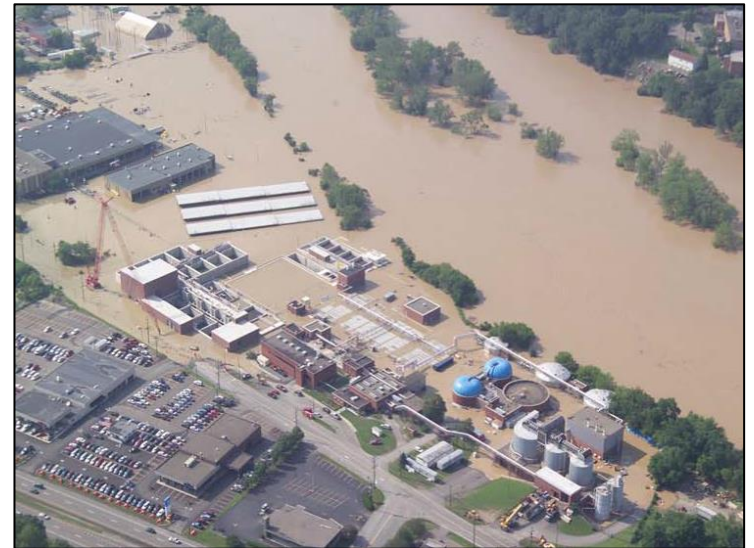
2006 Binghamton/Johnson City WWTTP
